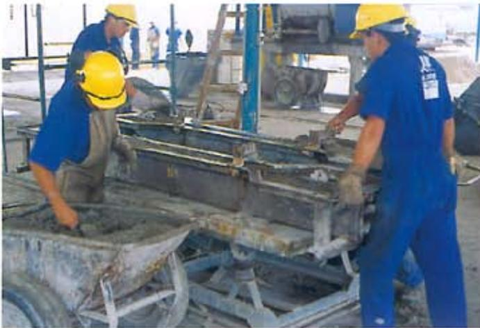
**Figuras 4.7 - Argamassagem**
